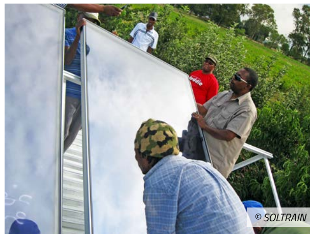
Lesotho practical training, installation of collectors.
