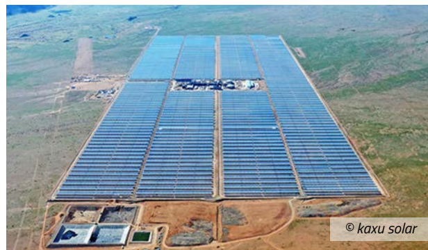
KaXu Solar One is South Africa's first concentrated solar power plant using parabolic trough technology.
